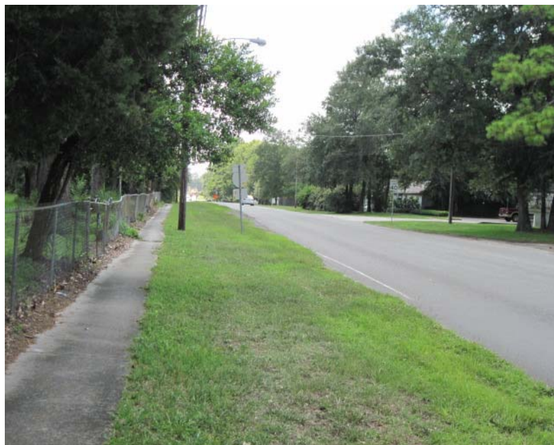
View off right-of-way looking north from subject property
